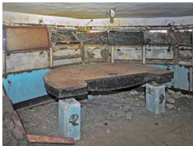
Fire Control South: the iron casting is the baseplate for a rangefinder
